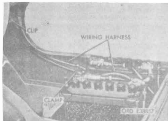
Figure 18-116. Crew compartment wiring and clips.
